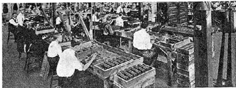
Fig. 23.—Assembling Telephone Ringers.
