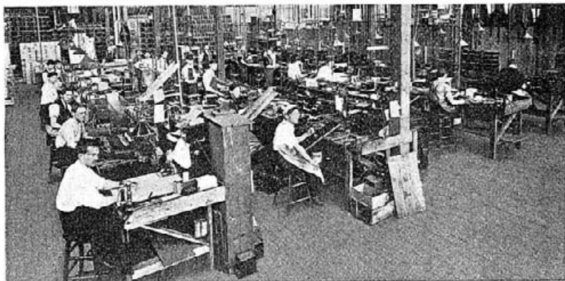
Fig. 29.—Assembling and Adjusting Receivers.
